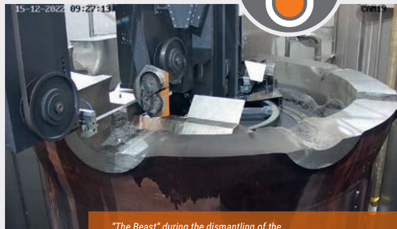
“The Beast” during the dismantling of the RPV flange area in the KKU.
