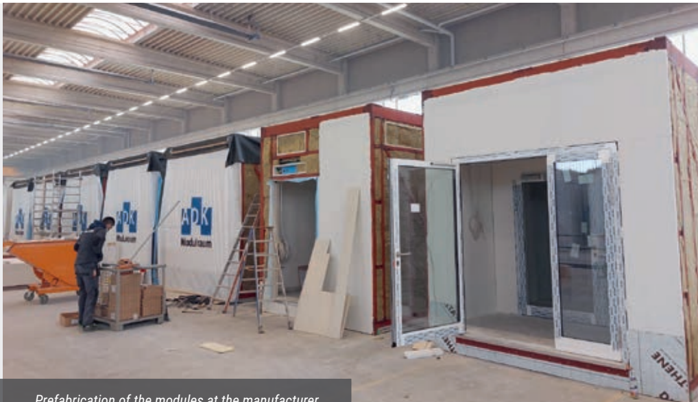
Prefabrication of the modules at the manufacturer.
