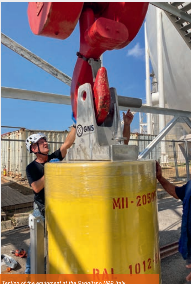
Testing of the equipment at the Garigliano NPP, Italy.
