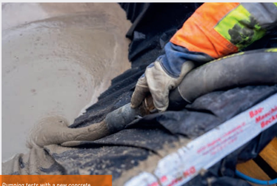
Pumping tests with a new concrete.
