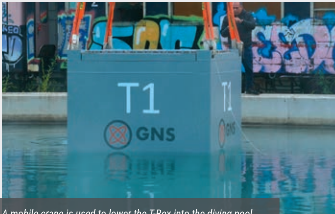
A mobile crane is used to lower the T-Box into the diving pool.
