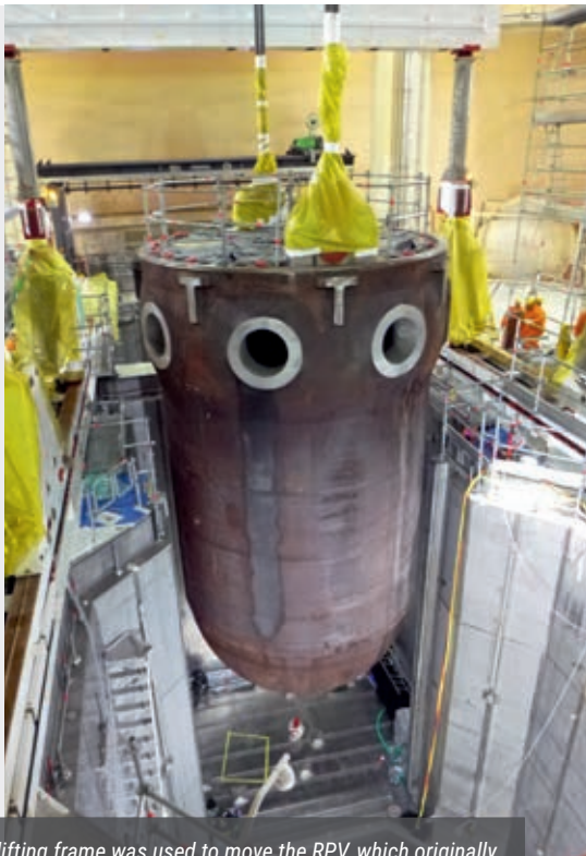
The Mammoet lifting frame was used to move the RPV, which originally weighed 530 t, onto the dismantling frame for the calotte.
