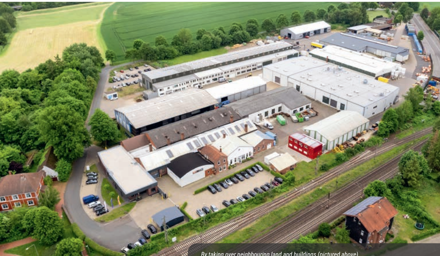
By taking over neighbouring land and buildings (pictured above), the area of EWB's headquarters in Bassum has almost doubled.
