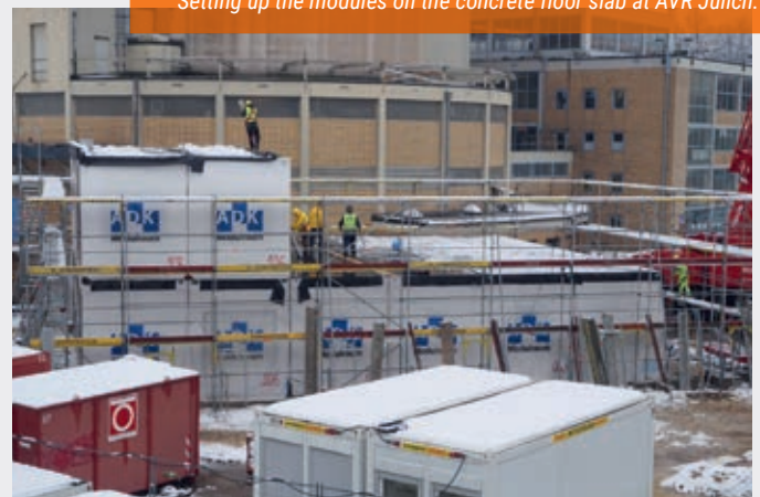
Setting up the modules on the concrete floor slab at AVR Jülich.
