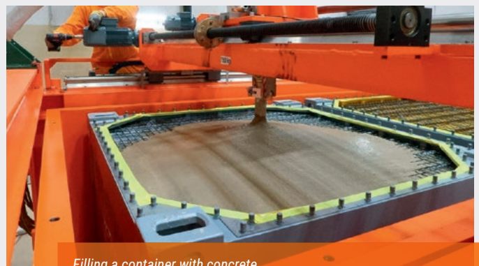
Filling a container with concrete.
