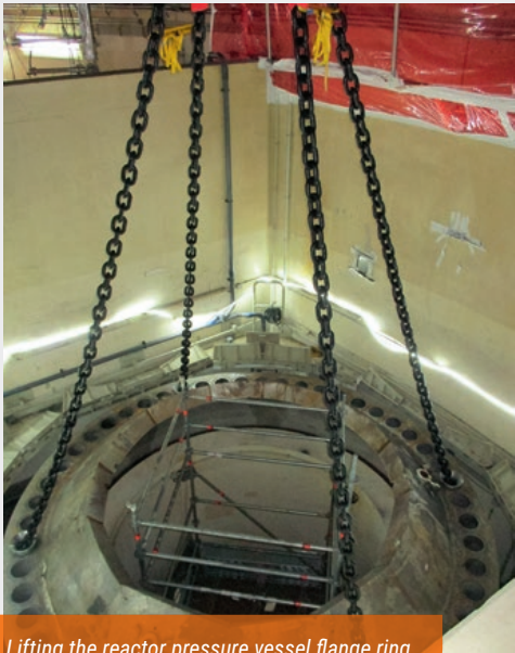
Lifting the reactor pressure vessel flange ring.
