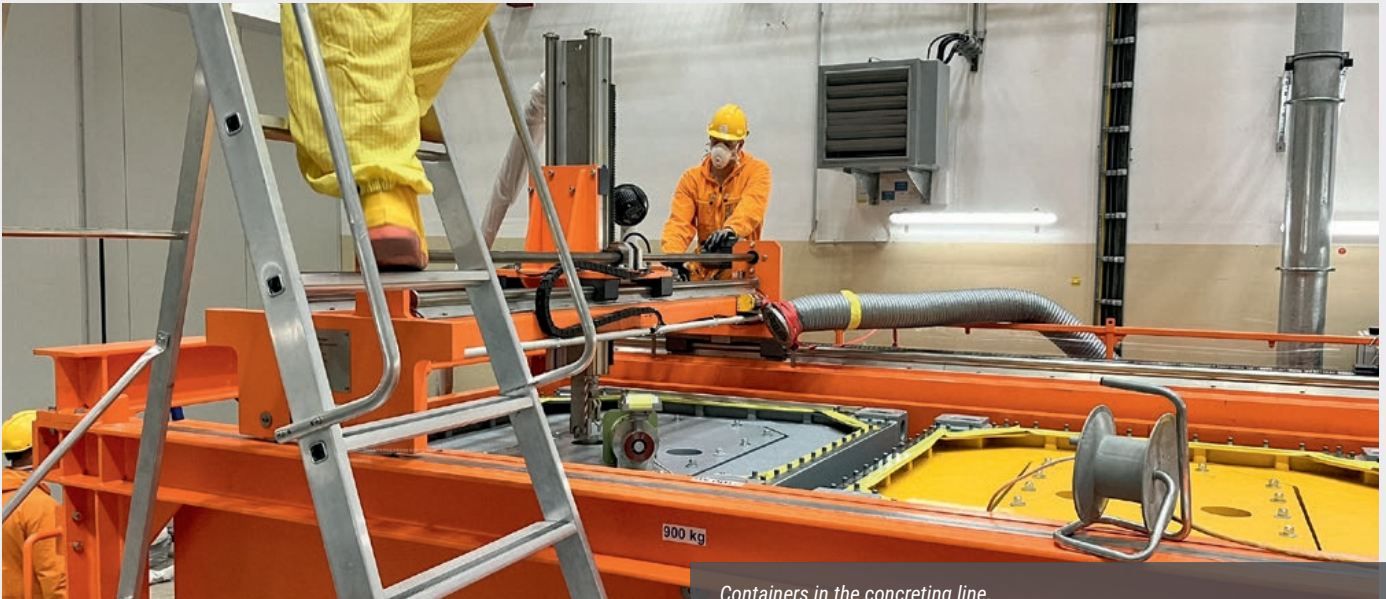
Containers in the concreting line.
