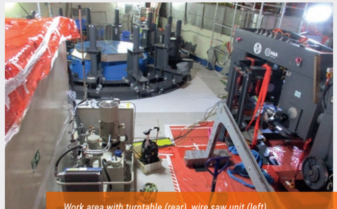
Work area with turntable (rear), wire saw unit (left), and band saw module (right).
