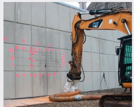
Test field for milling trials on a concrete wall using the newly developed milling method.
