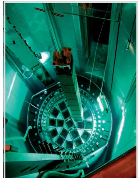
Fig. 1. Loading of a CASTOR<sup>®</sup> V/19 for PWR fuel assemblies.
