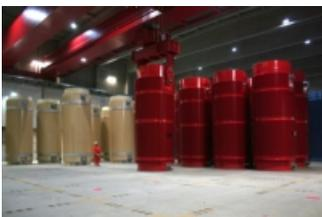
On a floor space of approx. 5,000 m<sup>2</sup>, TBL-G offers 420 storage positions for transport and storage casks for spent fuel and HLW.
