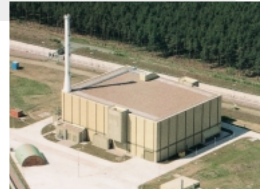
PKA construction site on the BLG premises
