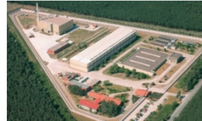
BLG site with the transportation cask storage facility
