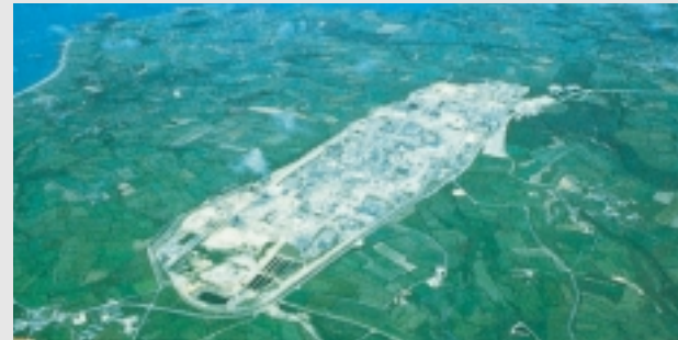
Plant in La Hague
